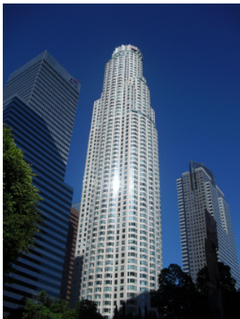
U.S. Bank Tower – CBM's office at 51st floor
